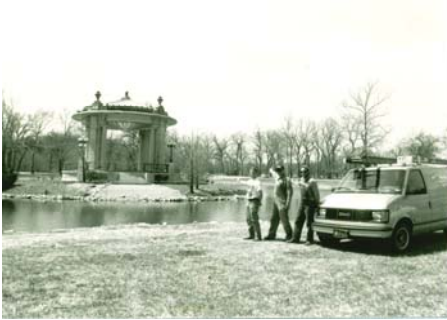
Forest Park Renovation Project 1992
